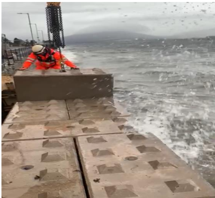
Ardbeg sea wall defences.
